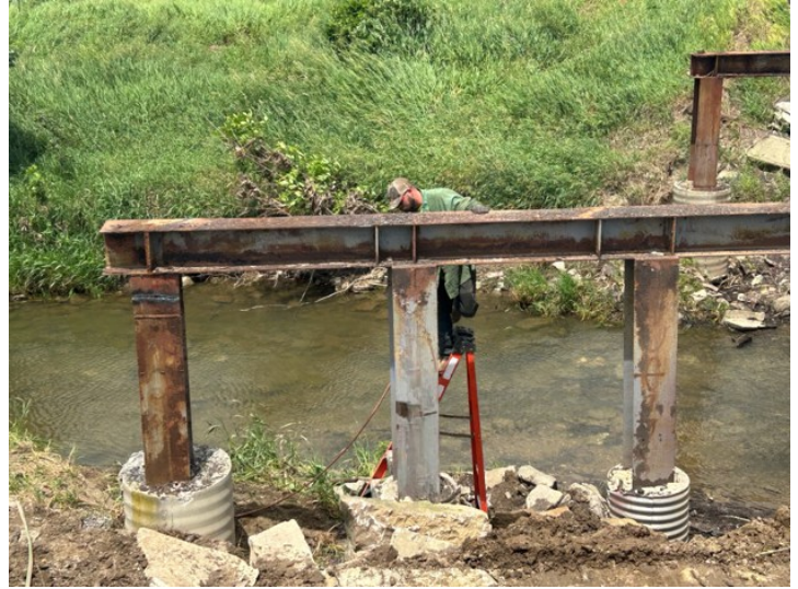
Dan Johnson working on getting the piers out CR 39 bridge replacement working on
