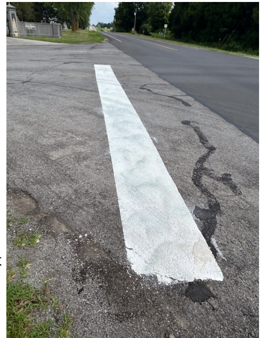
Stop bar painted on County Road 37
