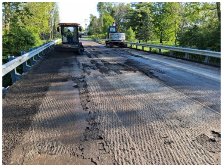
Milling on County Road 130
