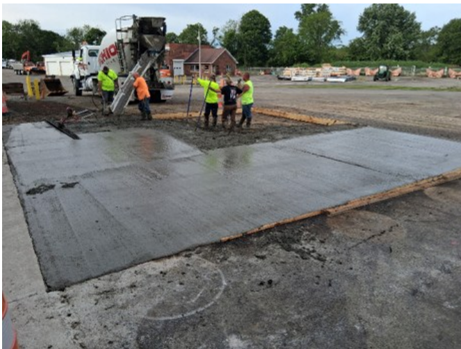
Bridge crew working on the cement pad at the LCEO compound
